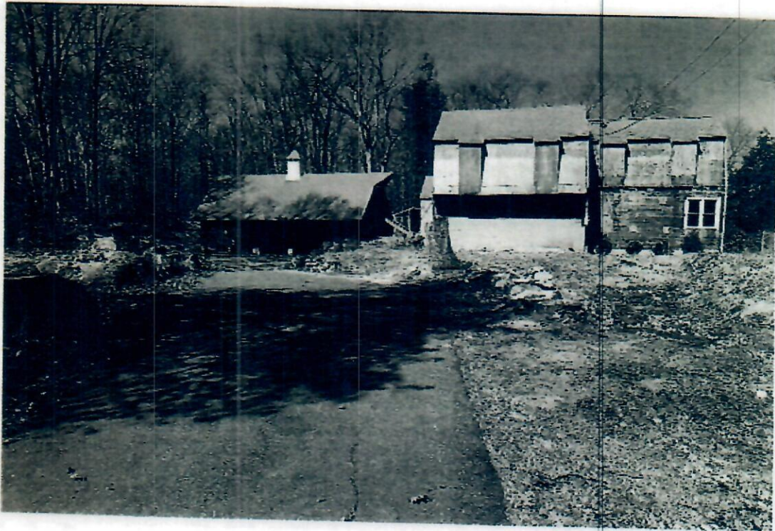
Photo 2 Looking north along driveway and toward residence and detached garage. April 2019- The 4 Ledgewood Place, LLC Site, 4 Ledgewood Place, North Castle, NY
