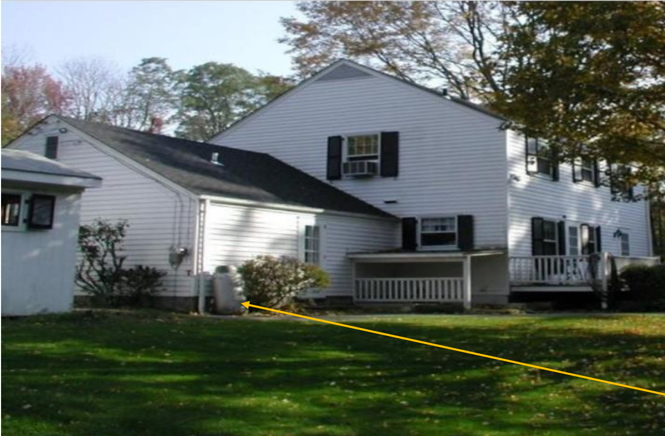
Current location of Propane tank
