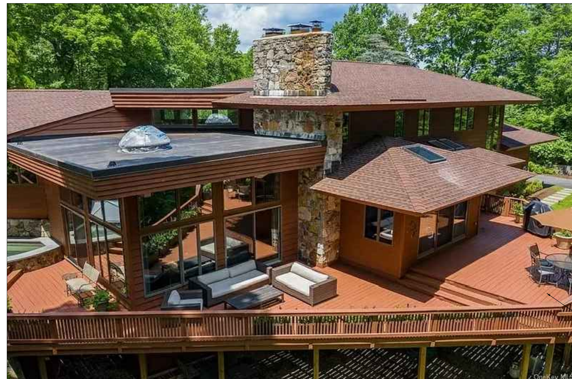
3 PHOTO OF DECK TO BE DEMOLISHED SCALE: N.T.S.
