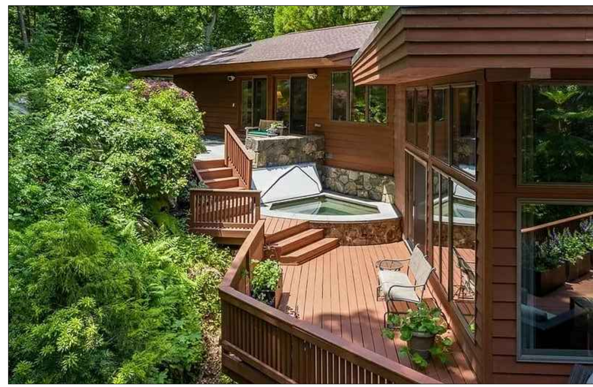
1 PHOTO OF DECK TO REMAIN SCALE: N.T.S. BEYOND THIS POINT KEEP EXISTING DECK FRAMING AND REPLACE HANDRAILS AND DECK BOARDS
