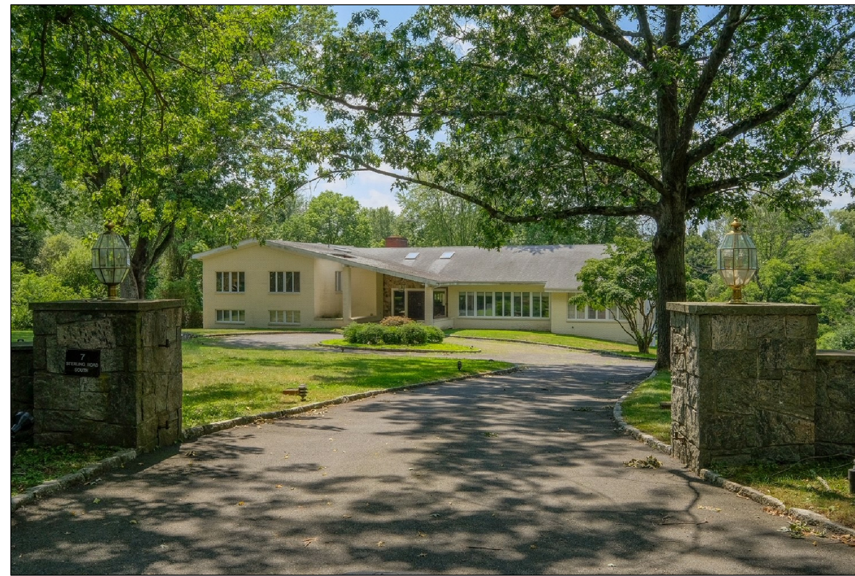
EXISTING FRONT ELEVATION FROM ROADWAY
