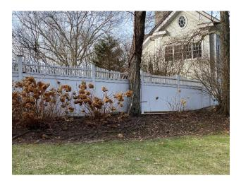
B. Wooden post and split rail around back of property. Below is a photo of part of this fence (current). This will be replaced with an identical new fence, 4 feet tall, with posts set in concrete (and with wire). Linear length is 560 ft in total. There are a total of 5 gates in this fence, which will also be replaced with self closing and latching hardware.
