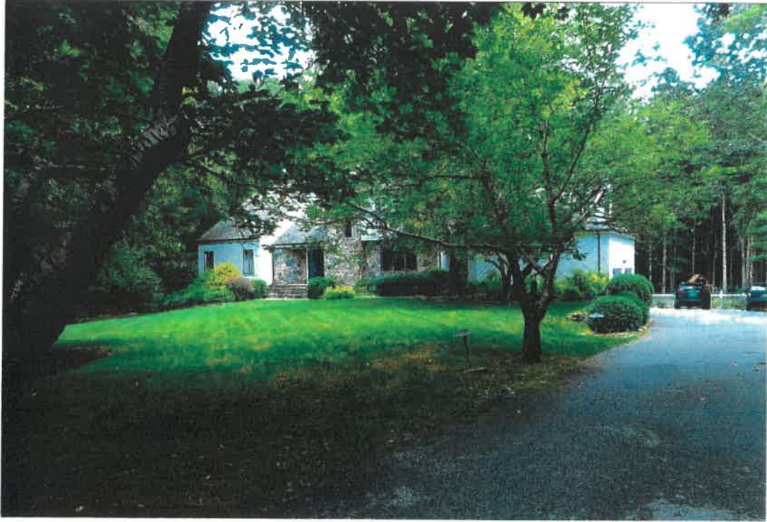
Photo 1 Looking east long the beginning of the driveway and toward the residence.
