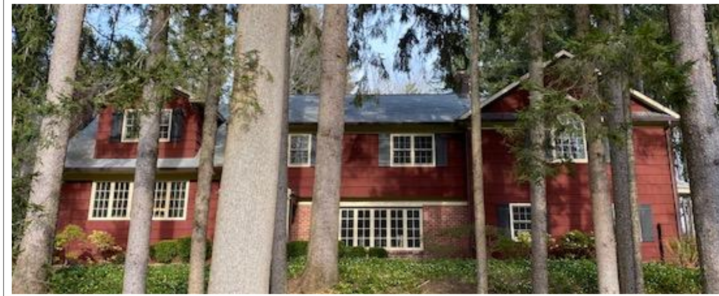
CLOSE VIEW OF EXISTING FRONT ELEVATION
