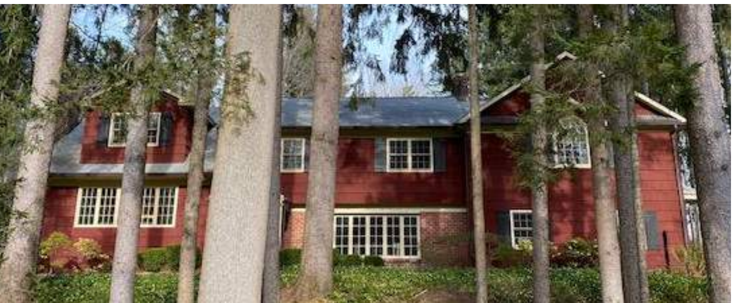
CLOSE VIEW OF EXISTING FRONT ELEVATION
