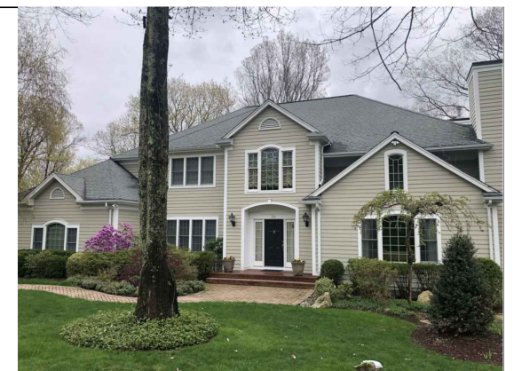
PICTURE OF EXISTING HOUSE (FRONT/WEST)
