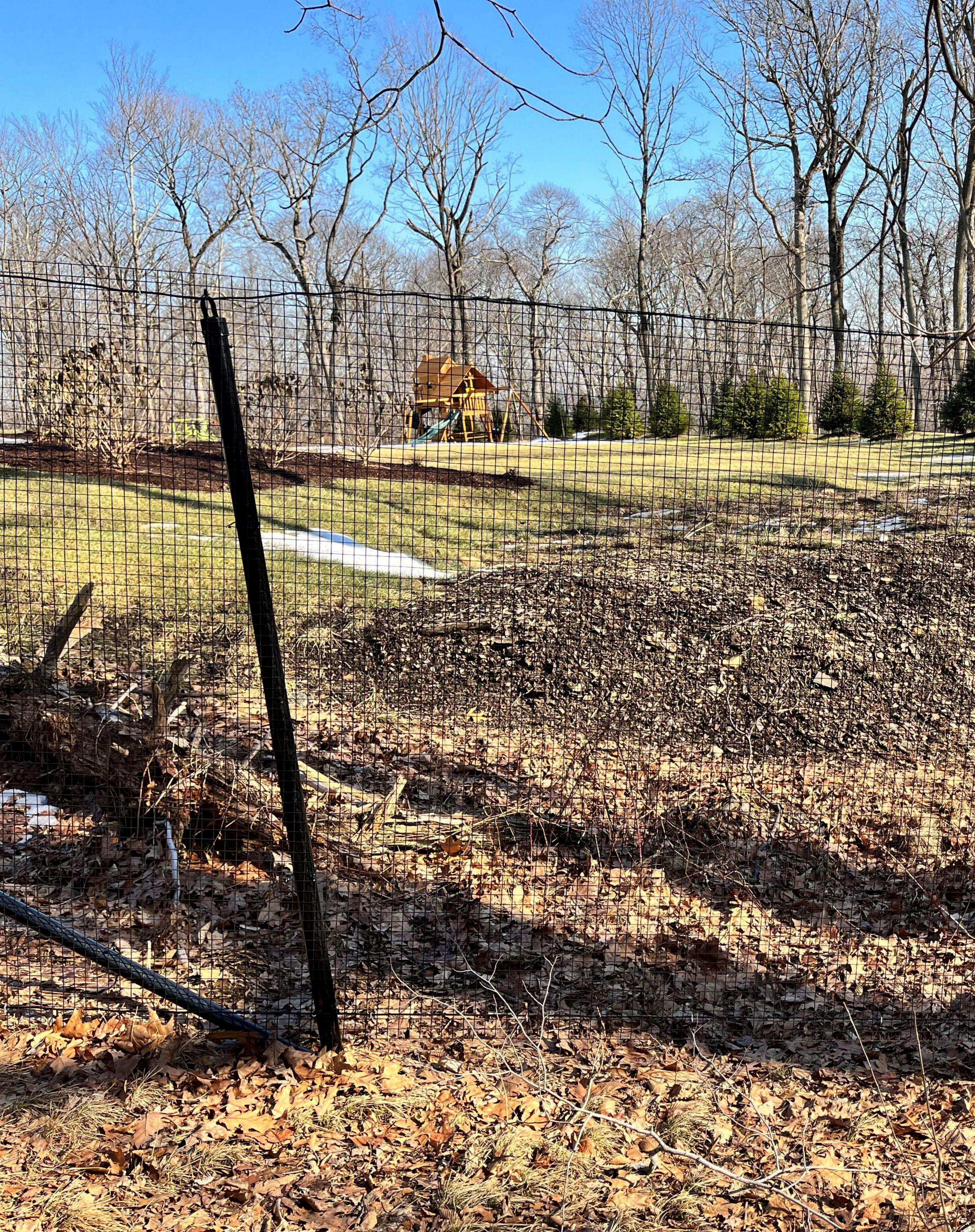
6 FT TALL DEER FENCE with heavy duty steel posts painted black, poly **Covered wire mesh with 1"x1" Openings. Footings will be min 2'6**" into the ground and embedded in **Quickrete concrete.** Tension wire (poly coated as well) on top and bottom. All corner posts will have **diagonal bracing**
