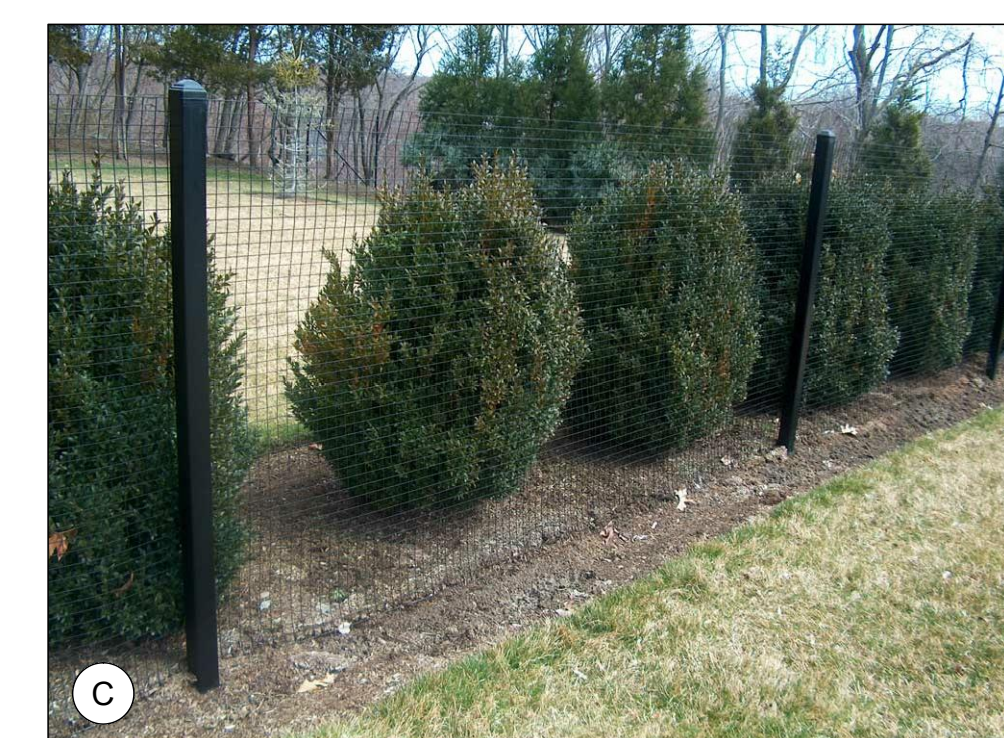
C WELDED WIRE DEER FENCE OR BLACK VINYL COATED CHAIN LINK FOR RUNS NOT ATTACHED TO HOUSE
