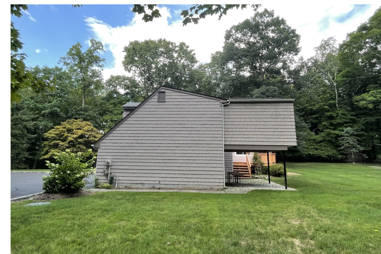
EXISTING VIEW RIGHT SIDE ELEVATION
