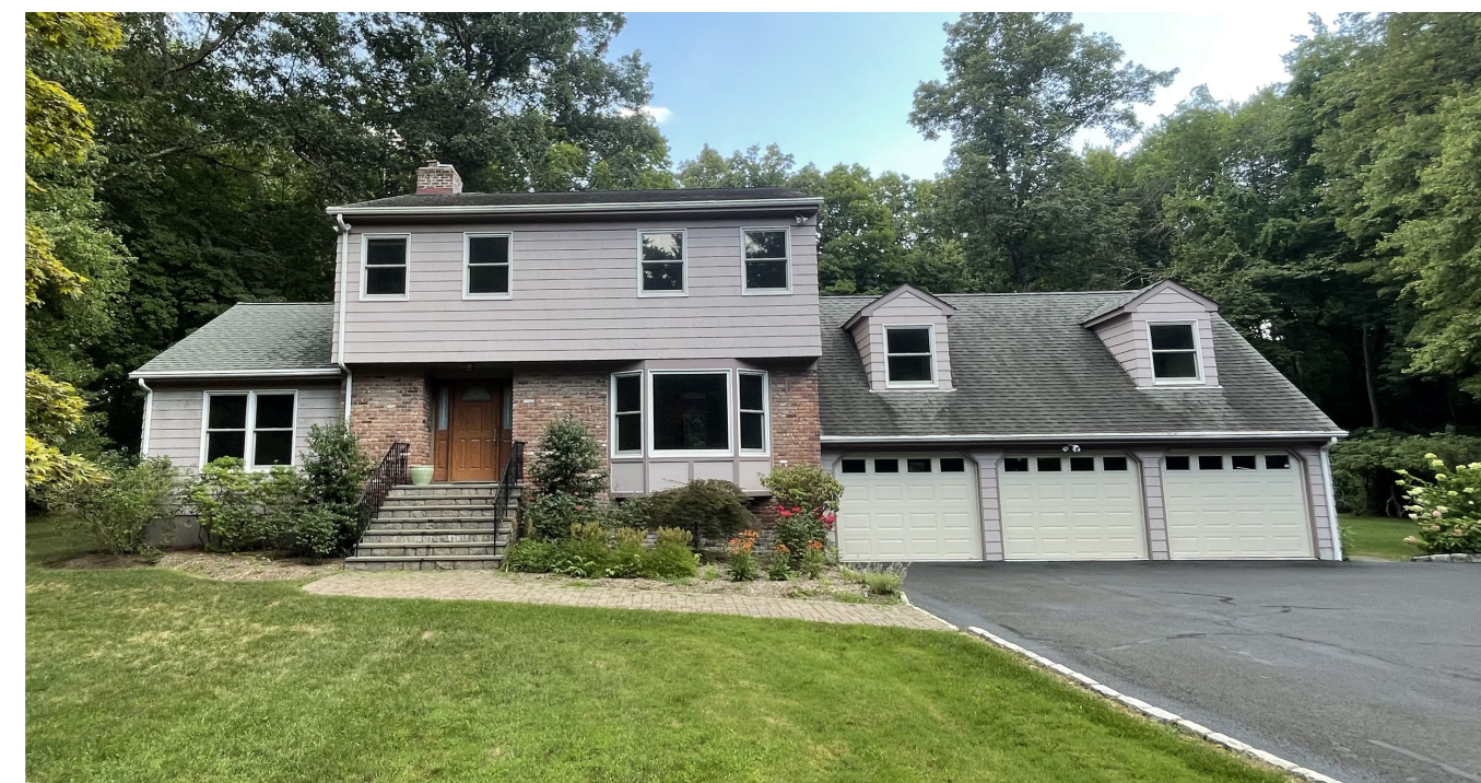
EXISTING VIEW OF FRONT ELEVATION
