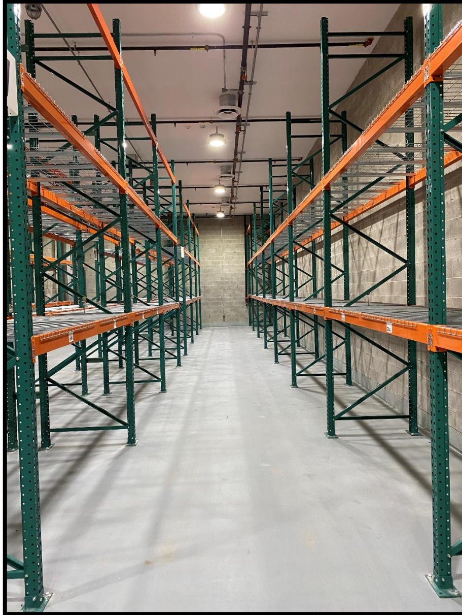
Photograph of recently constructed proposed storage area for additional chemical compounds.
