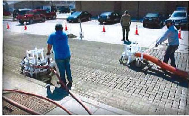
Figure 24. This equipment blows sediment and soiled aggregate from the joints and uses vacuum equipment to remove them.
