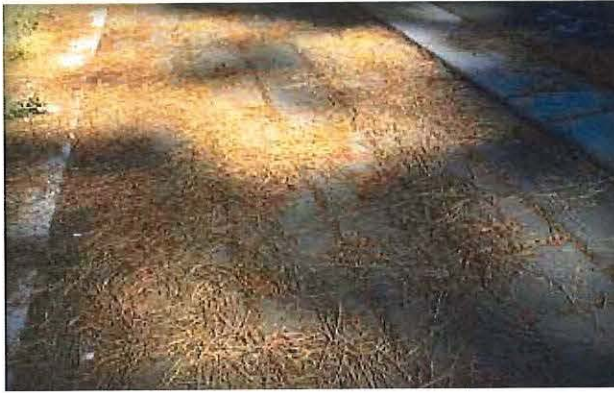
Figures 7 and 8. Pine needles and leaves eventually will degrade and get compacted into the joints from traffic. They should be removed by sweeping or vacuuming before that happens.
