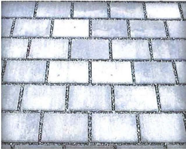
Figure 4. Keeping PICP joints filled with permeable aggregate facilitates removal of accumulated sediment.
