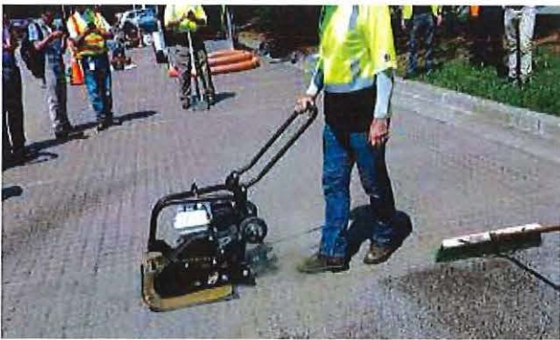
Figure 25. No matter the equipment used, after removing sediment soiled aggregate, clean aggregate is placed in the joints, the surfaced cleaned and compacted.
