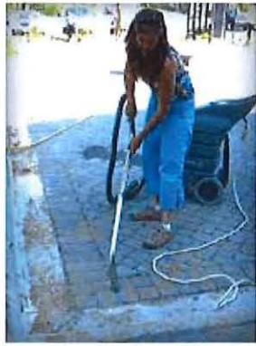
Figure 17. Wet/dry shop vacuum cleans loose sediment from a PICP residential driveway
