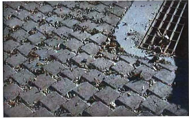
Figures 7 and 8. Pine needles and leaves eventually will degrade and get compacted into the joints from traffic. They should be removed by sweeping or vacuuming before that happens.
