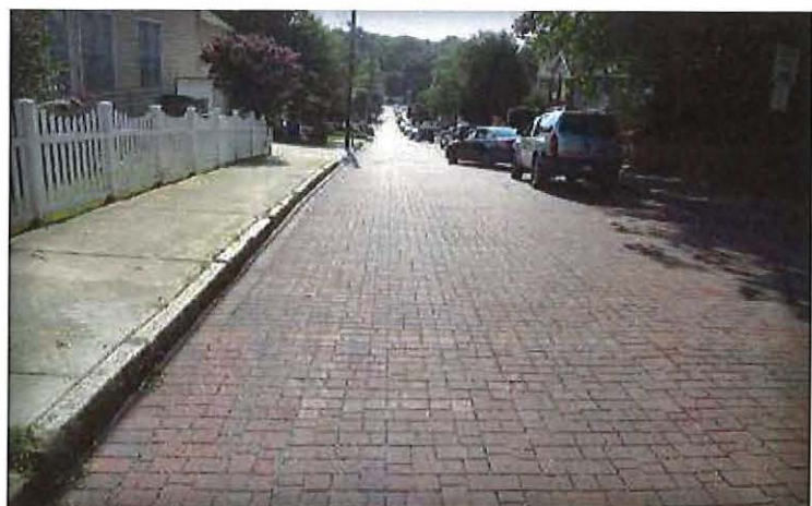
Figure 1. PICP is seeing increased use in municipal streets to reduce stormwater runoff, local flooding, storm pipe upsizing, and combined sewer overflows. These streets are in Atlanta, GA.
