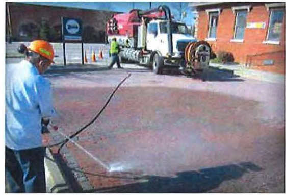
Figure 19. Power washing requires a little practice to minimize jointing stone removal.
