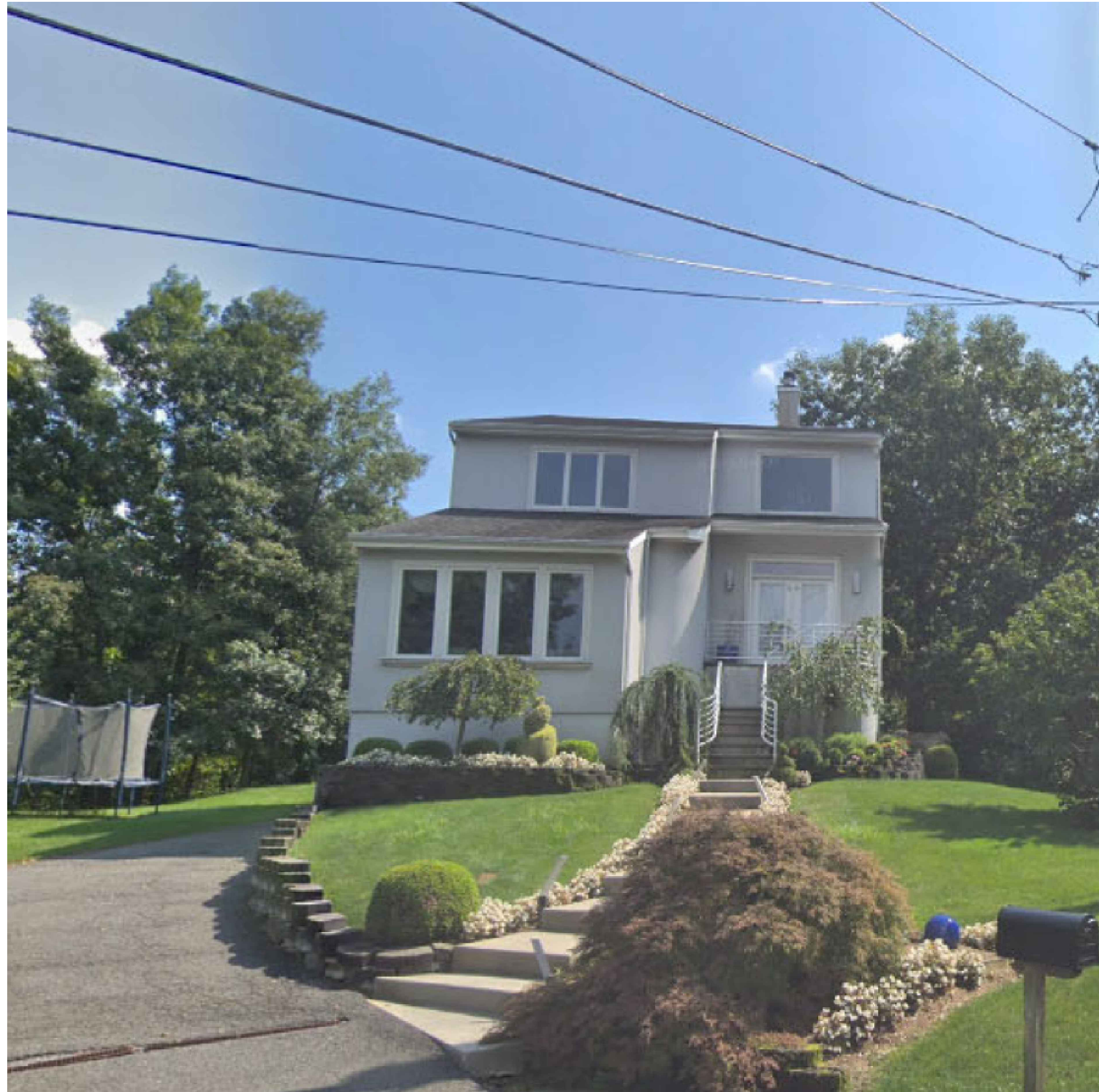
20 NETHERMONT AVE SINGLE FAMILY RESIDENCE
