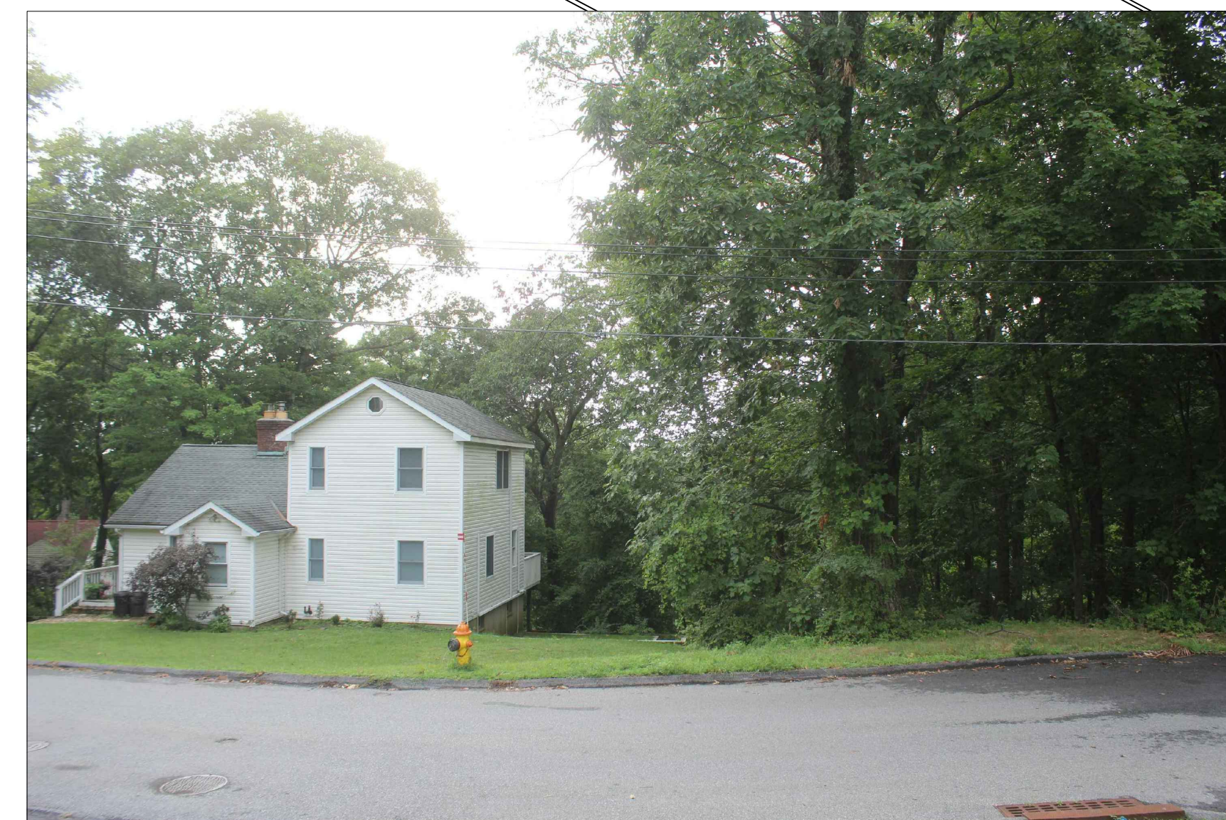
19 NETHERMONT AVE SINGLE FAMILY RESIDENCE
