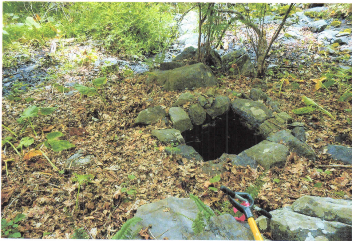
Photo 10 Looking southeast toward remains of fieldstone-lined well next to pump / well house and located next to southwest corner of the site.
