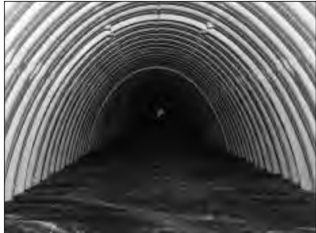
Looking down the Isolator Row.
