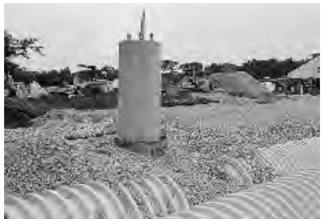
Figure 15 – Chamber bed placed around light post.
