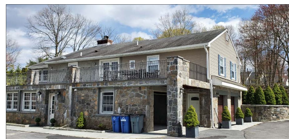
REAR VIEW FROM DRIVEWAY
