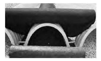
Inspection is easily accomplished through the upstream manhole or optional inspection ports. Maintenance of an Isolator Row is fast and easy using the JetVac process through the upstream manhole. Section 12.0 explains the inspection and maintenance process in more detail.
