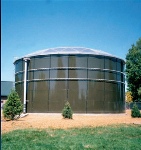
Ground Storage Tank
