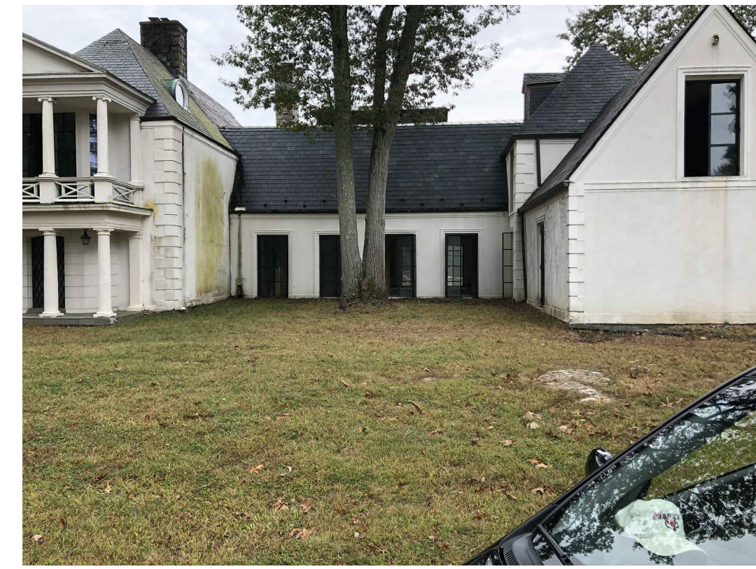
5 CLOSE UP VIEW OF FRONT (EAST) FACADE
