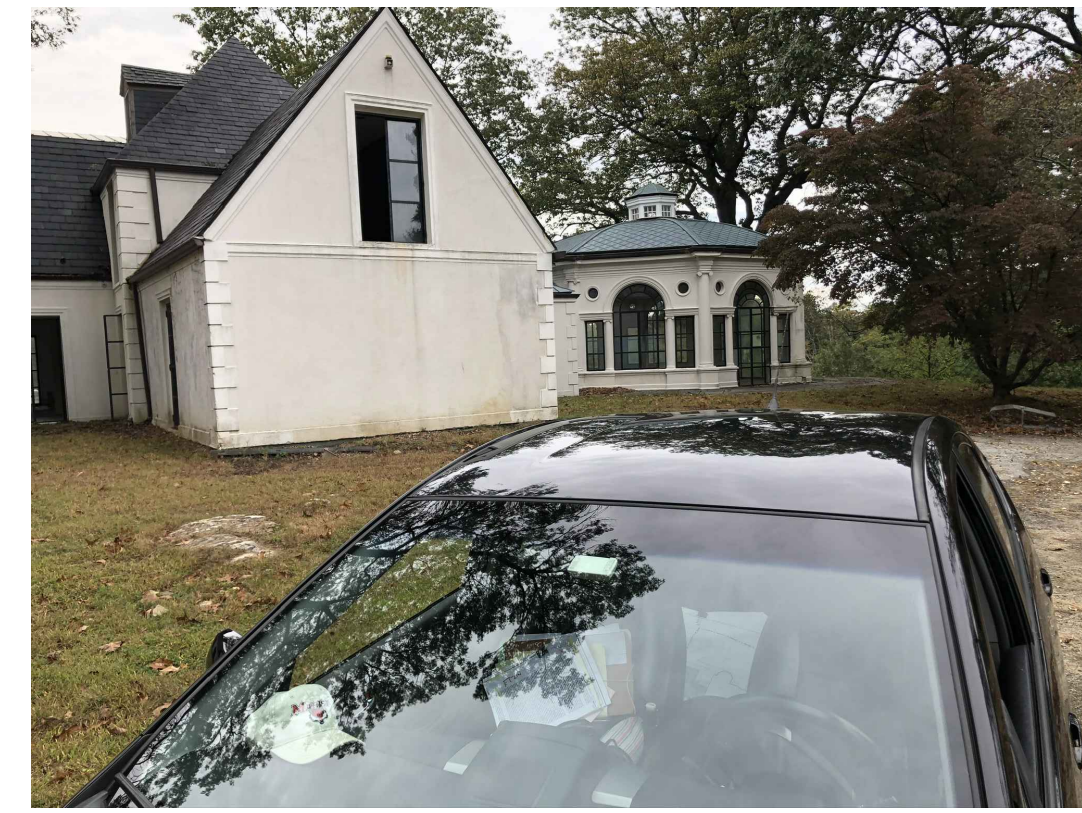
4 NORTHERN MOST EXTENSION OF FRONT (EAST) FACADE OF FORMER RESIDENCE
