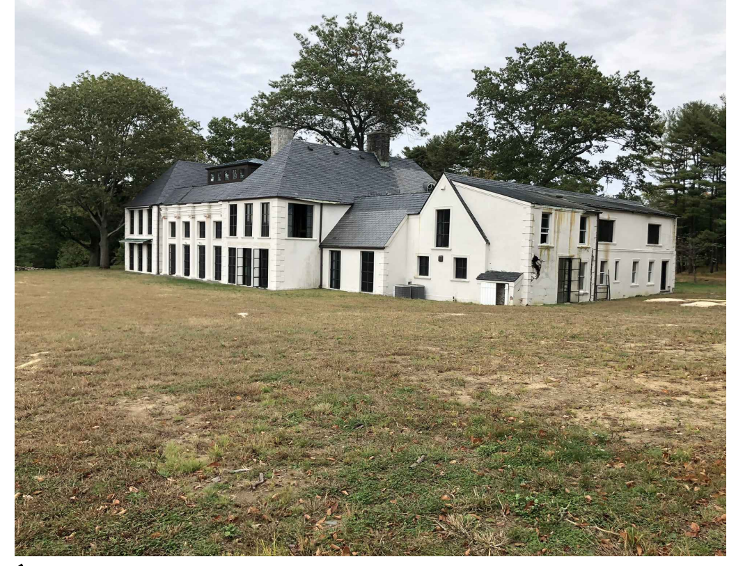
7 VIEW TO SOUTH WEST FACADE OF EXISTING MAIN STRUCTURE. NOTE THAT PORTION OF SOUTH WING (AT RIGHT OF PHOTO) IS TO BE REMOVED. NEW GARAGE ADDED TO SOUTH FACE OF HOUSE
