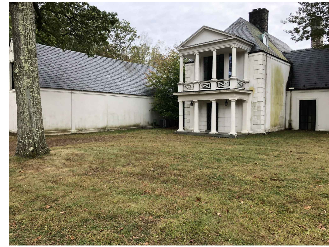
3 CLOSE UP VIEW OF ARCHITECTURAL DETAILS
