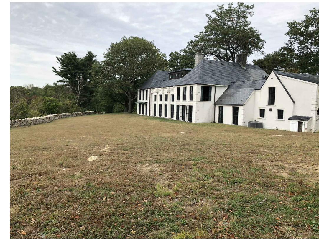
6 VIEW NORTH TO REAR OF ORIGINAL HOUSE. NOTE THAT YARD HAS BEEN LEVELED, SUPPORTED BY RETAINING WALL AT LEFT OF PHOTO
