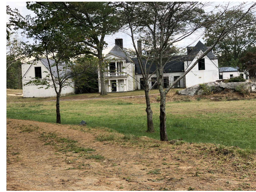
2 FRONTAL VIEW OF EAST FACADE OF ORIGINAL HOUSE
