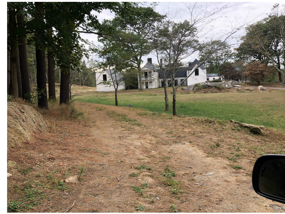
1 VIEW WEST OVER PROPERTY FRONT YARD TOWARD EAST FACADE OF EXISTING ORIGINAL MAIN HOUSE
