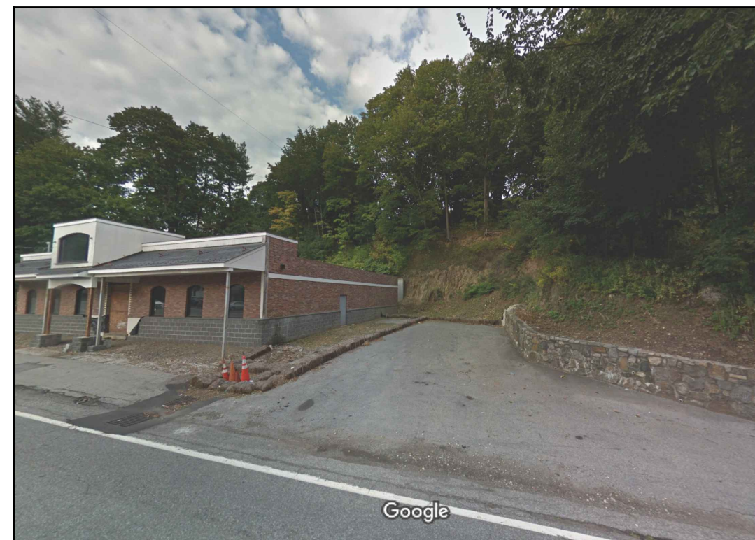
VIEW LOOKING UP SOUTHERN PROPERTY LINE
