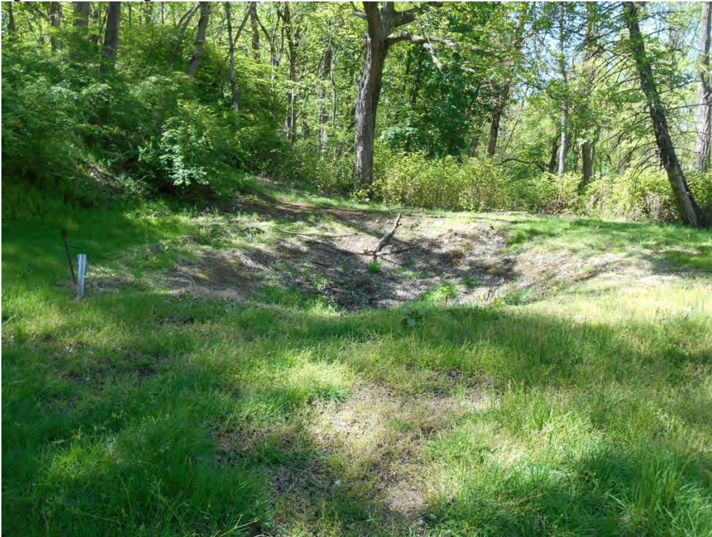
Photograph 16. The rear yard of the residence showing a large pit where a former water tank/tower was located. View looking south.
