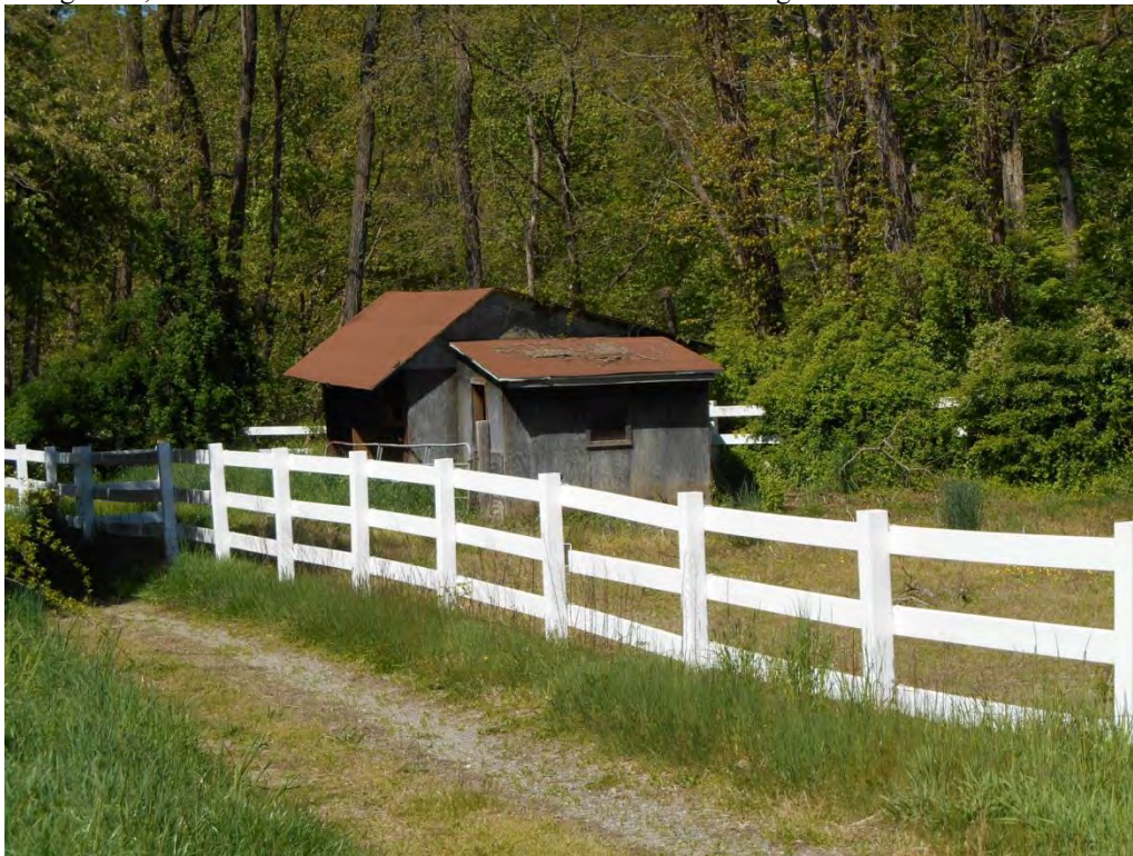
Photograph 8. An existing paddock with a one-story horse stall and shed, which is proposed to be demolished. View looking southwest.
