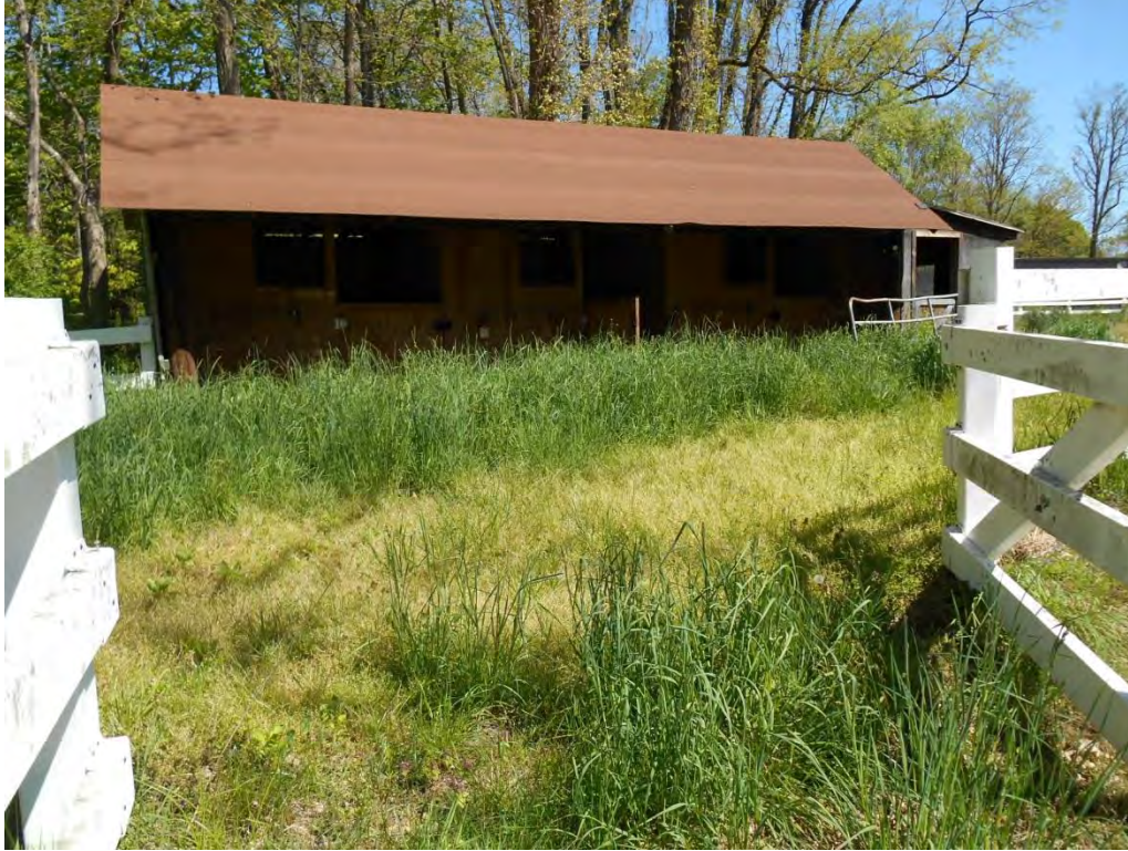
Photograph 9. Detail of the one-story frame horse stall and shed that is proposed to be demolished. View looking north.
