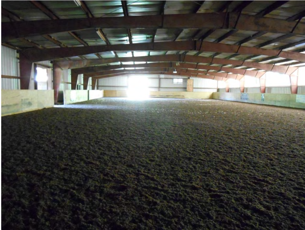
Photograph 5. The interior of the indoor riding arena. View looking southwest.
