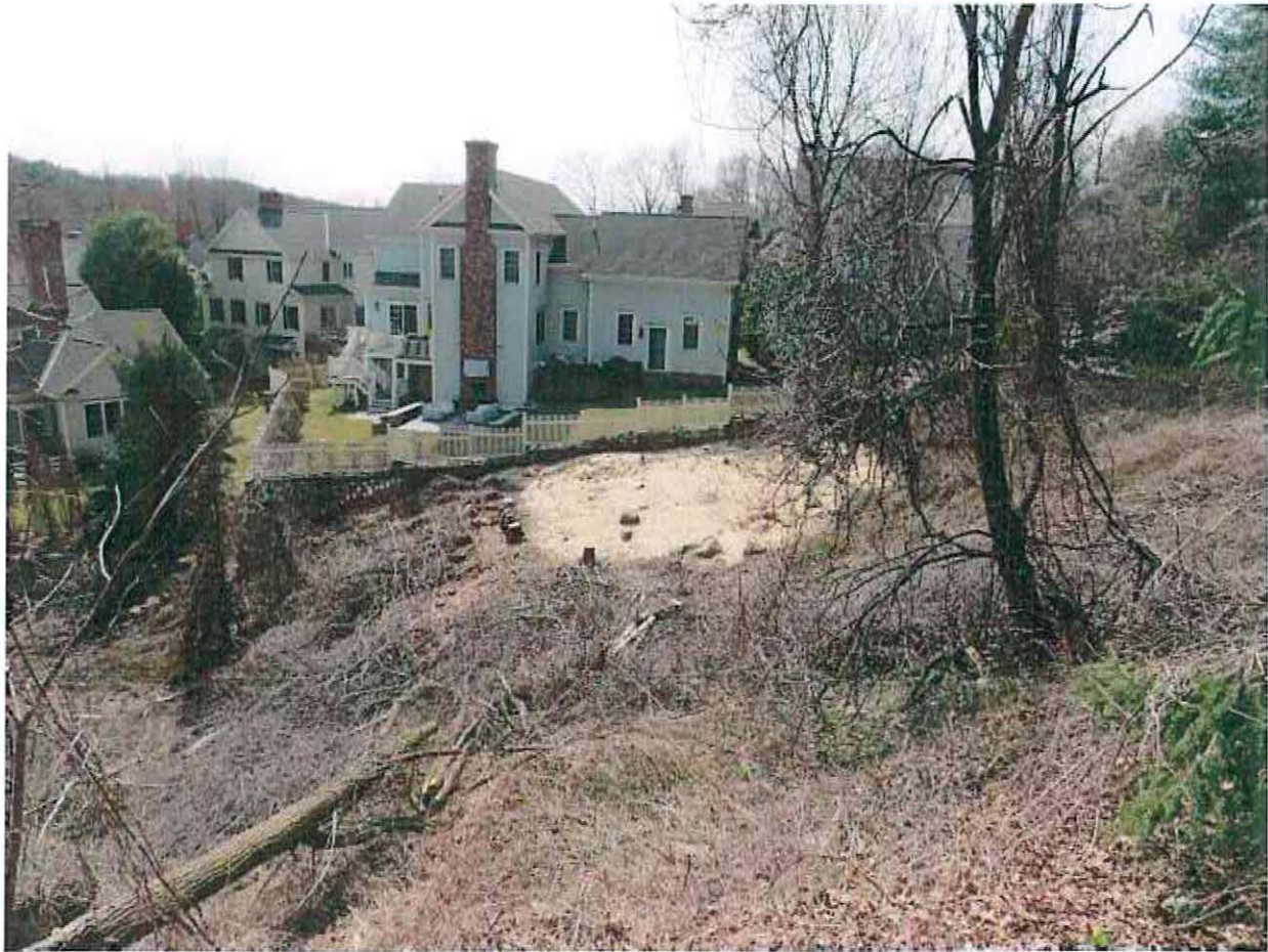
Photos 11-14 Taken By John Moran 3/23/21
