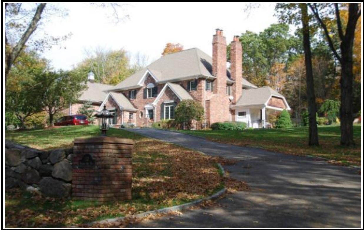
Photo 15: 10 Hidden Oak Road. House is recent construction. View to northwest.
