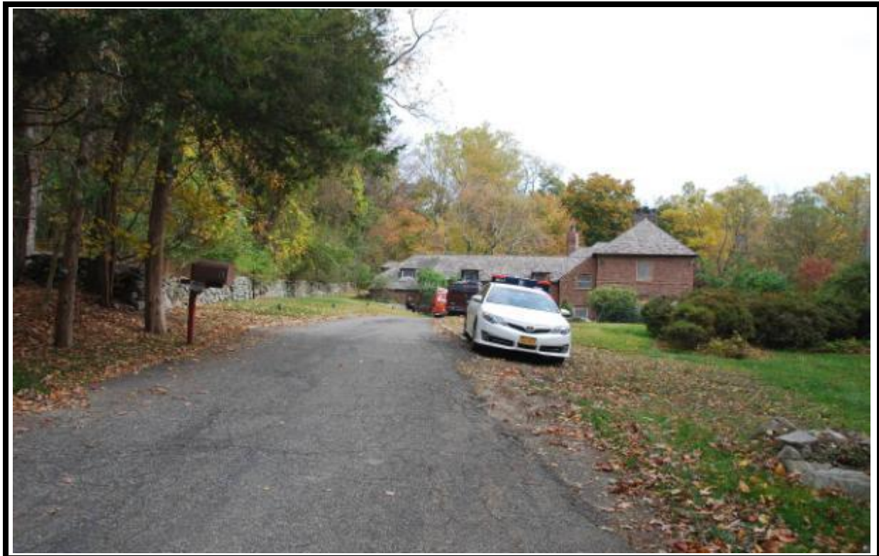
Photo 11: 6 Hidden Oak Road. House is currently under renovation. View to northeast.
