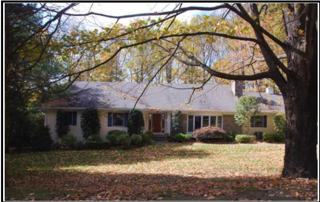
Photo 14: House located north of 5 Hidden Oak Road dates to 20 th century. View to east.
