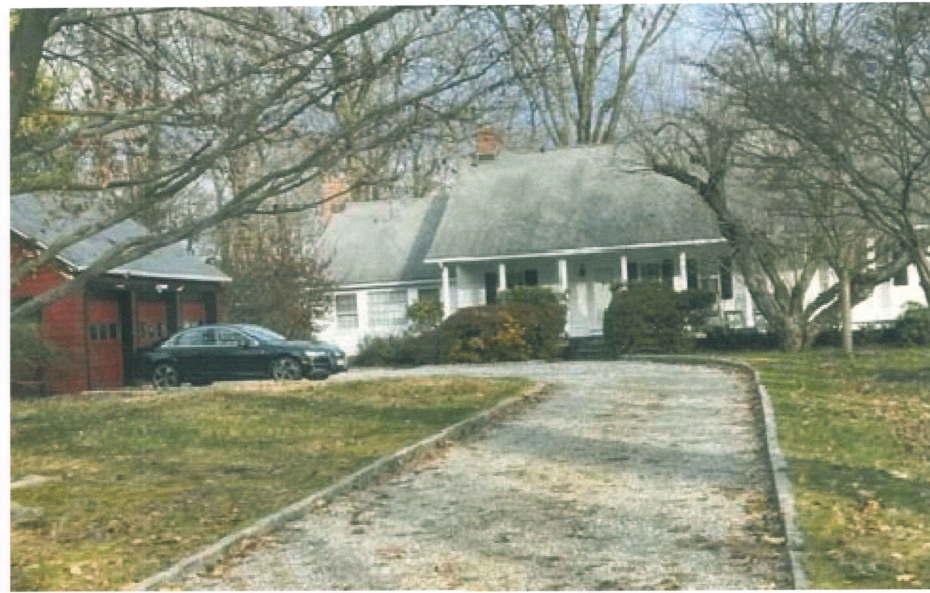
60 WHIPPOORWILL ROAD (ADJACENT LEFT)
