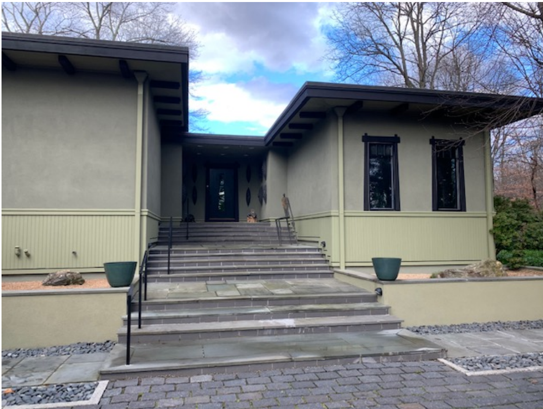
FRONT ENTRY OF EXISTING MAIN HOUSE
