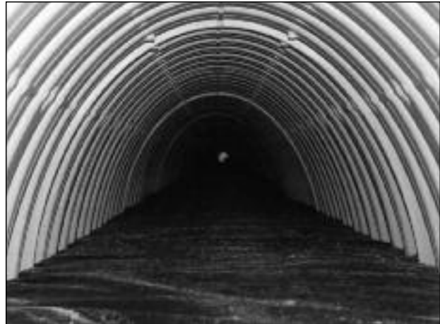
Looking down the Isolator Row.
