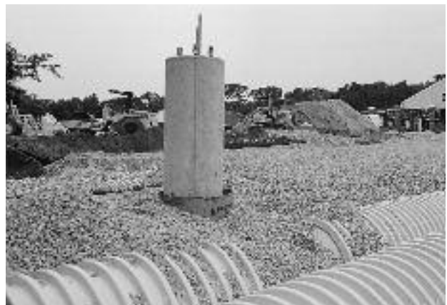
Figure 15 – Chamber bed placed around light post.
