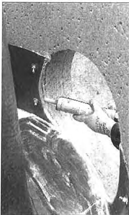
Fig 15. Seal inlet trough down the sides and along bottom of inlet coring with Sikaflex 1a sealant or equivalent.
