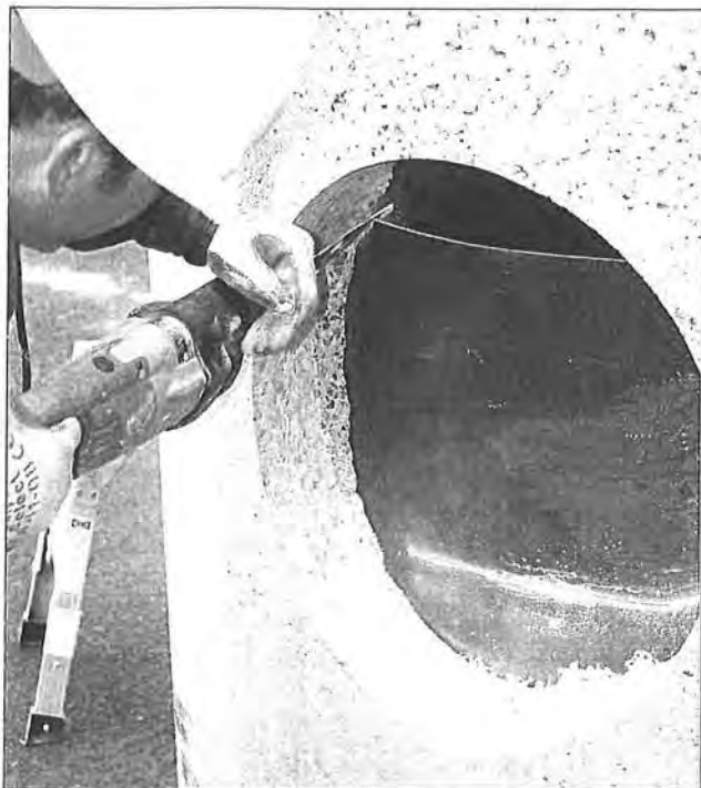
Fig 13. Remove trough flange blocking inlet coring.
