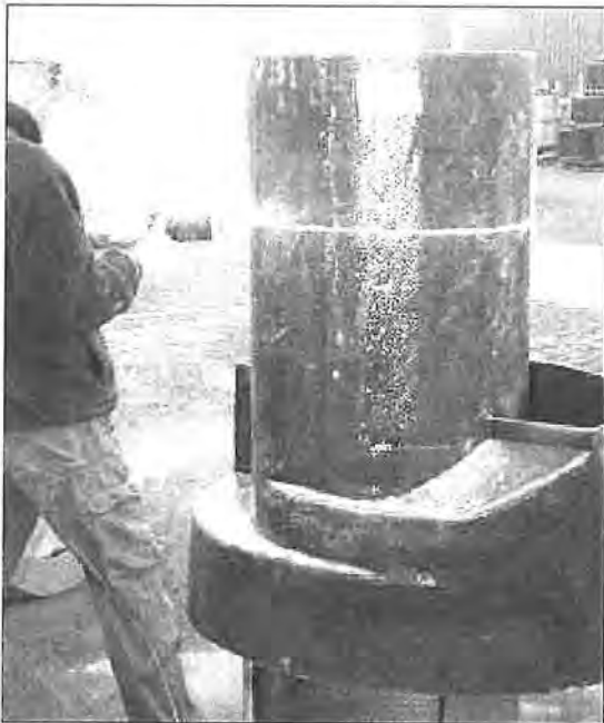
Fig 6. Removing top of inlet cylinder.
