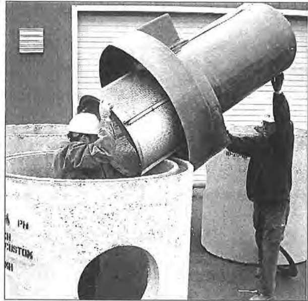
Fig 7. Lift inlet and screen assembly into manhole.
