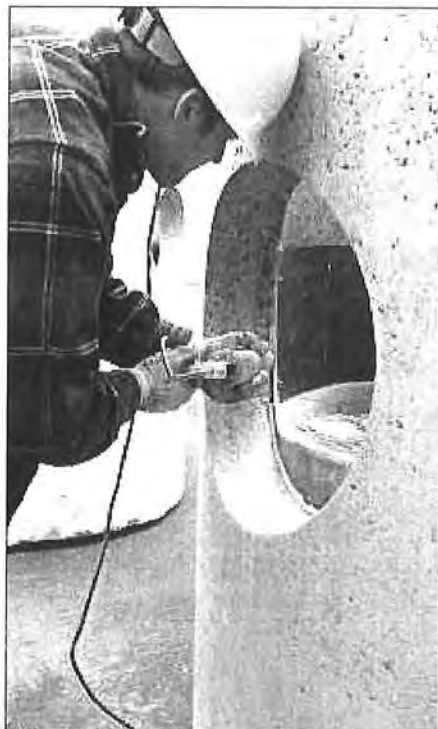
Fig 15. Seal inlet trough down the sides and along bottom of inlet coring with Sikaflex 1a sealant or equivalent.
