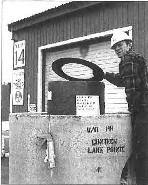
Fig 16. Installing PVC hydraulic shear plate.
