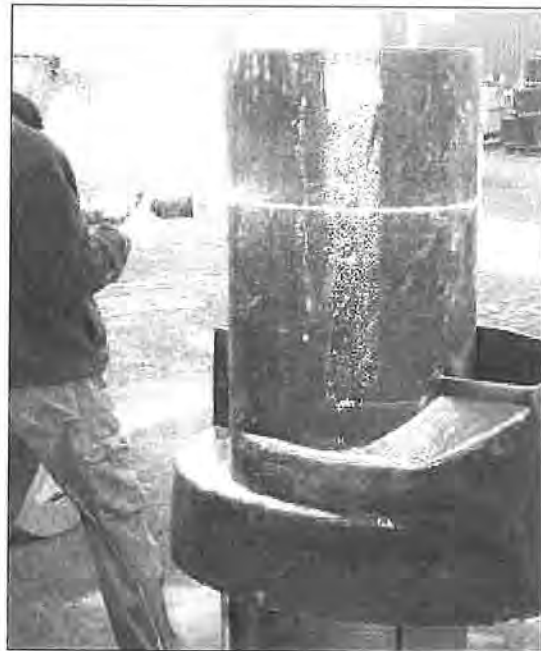
Fig 4. Attach screen to inlet with 1/2" bolts
