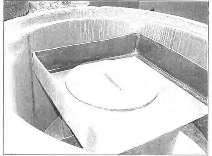
Fig 18. Deflector pan installed on top of cylinder.
