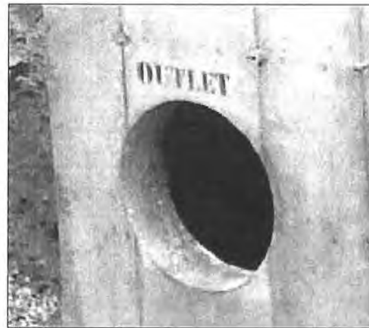
Fig 19. Stencil inlet and outlet coring.
