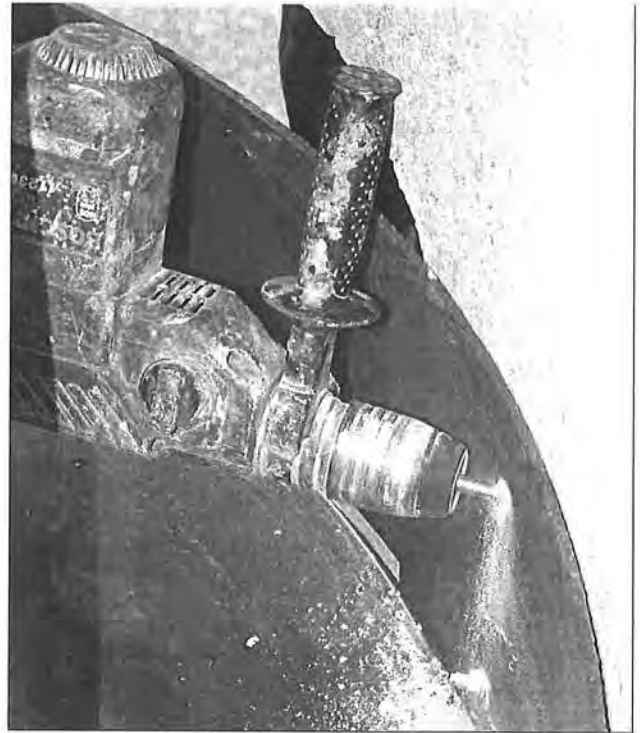
Fig 11. Drill concrete manhole for wedge anchors.
