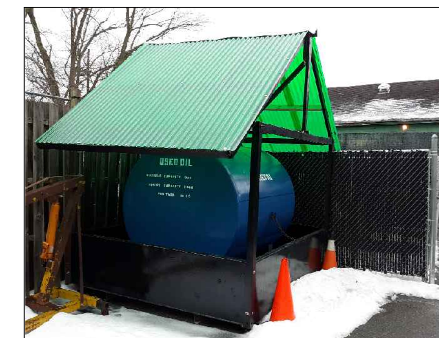
PHOTO 2 : EXISTING USED OIL STORAGE TANK WITH COVER.
