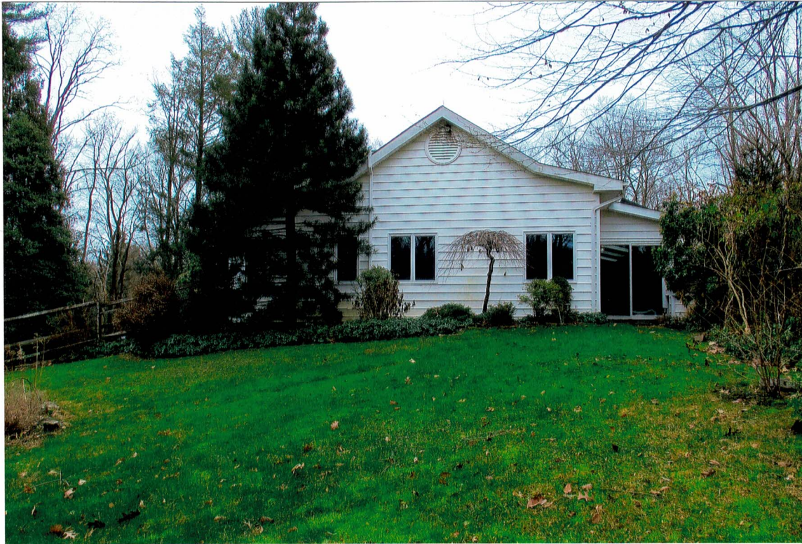
Photo 4 Looking southeast toward northwest side of residence.
