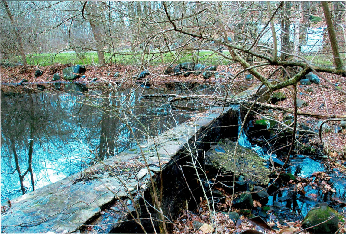
Photo 11 Looking southwest across dam of pond associated with wetland WL-“B”.
