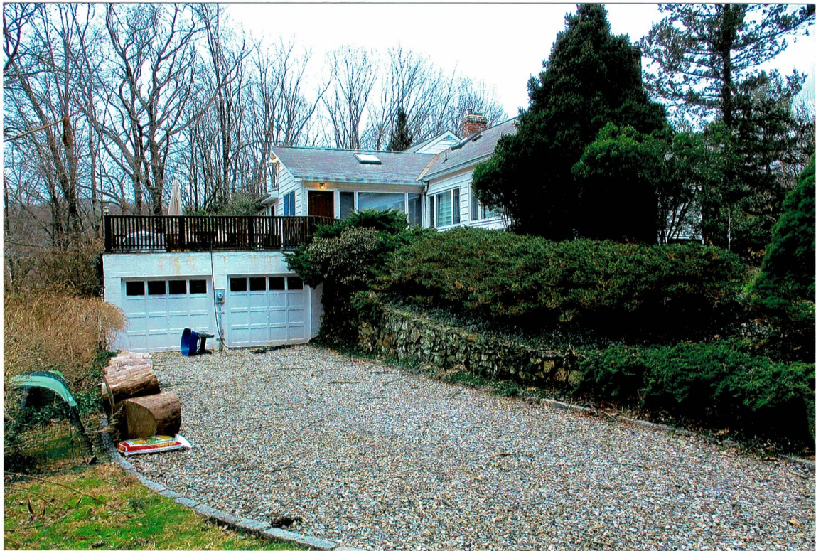
Photo 2 Looking northwest along driveway spur leading to south side of residence.
