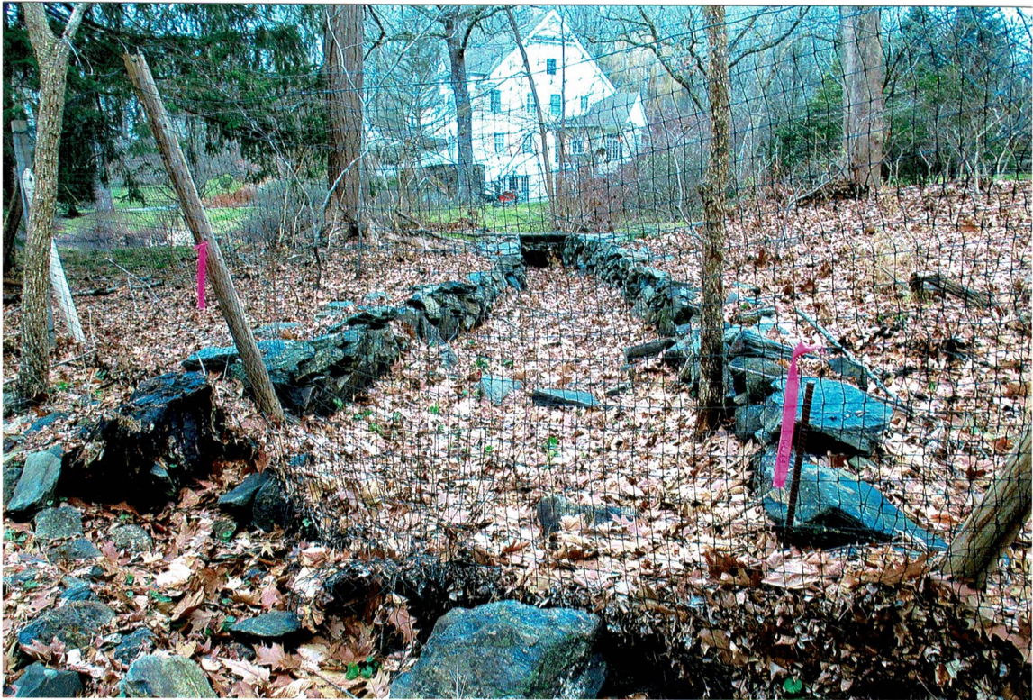
Photo 9 Looking southwest and upstream along stone-lined spillway channel connected to neighbor's pond that drains into brook associated with wetland WL- "A".
