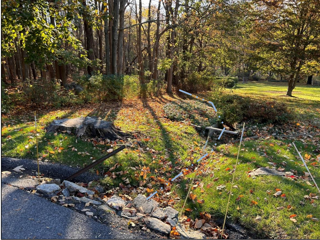
Photo 17. Looking southwest from 89/91 Byram Ridge Road where a Town drainage feature channels water towards the subject site. Shown by dashed line.
