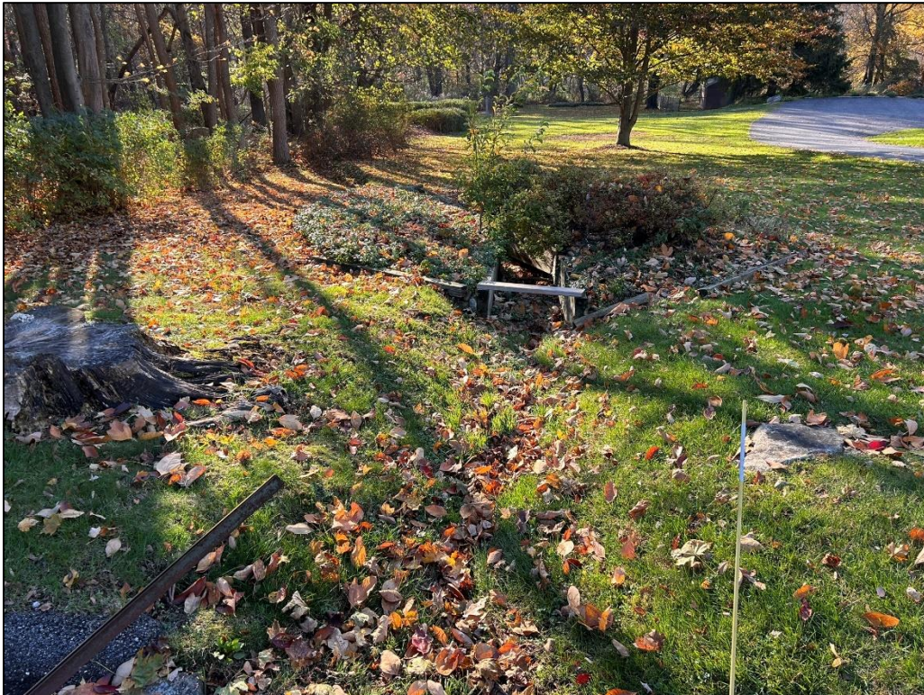
Photo 18. Another photo of the same drainageway which is shown channelized by wooden walls.
