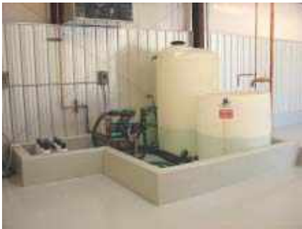
360 gallon open top mix tank with jet agitation and 750 gallon storage tank for rinsate or second mix tank
